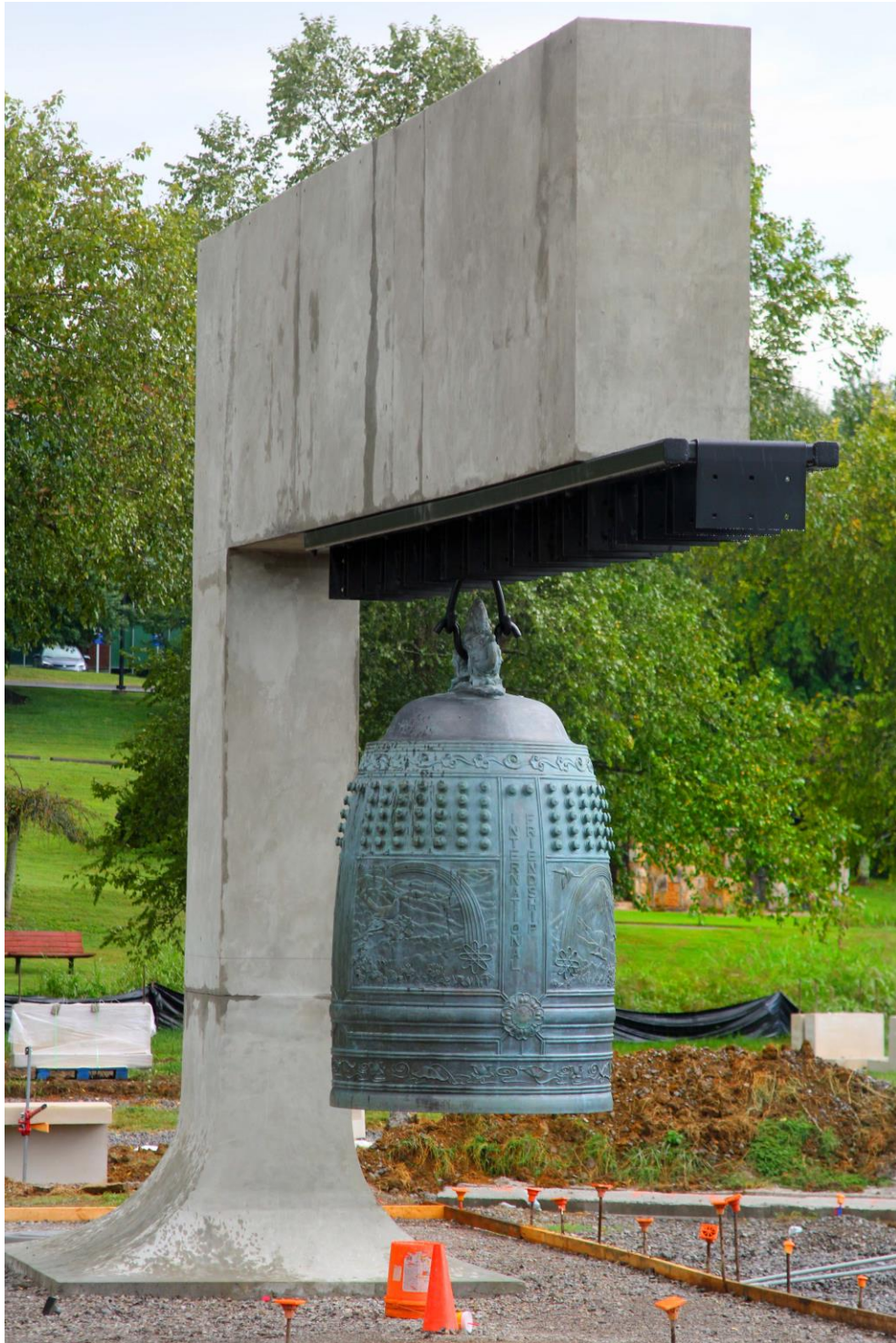
The Oak Ridge International Friendship Bell is hanging on the cantilever design bell support structure. The first step in a series of additional elements to be added to complete the Peace Pavilion.
